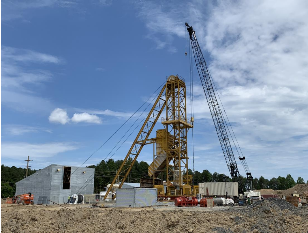
Service shaft construction headframe & support facilities
