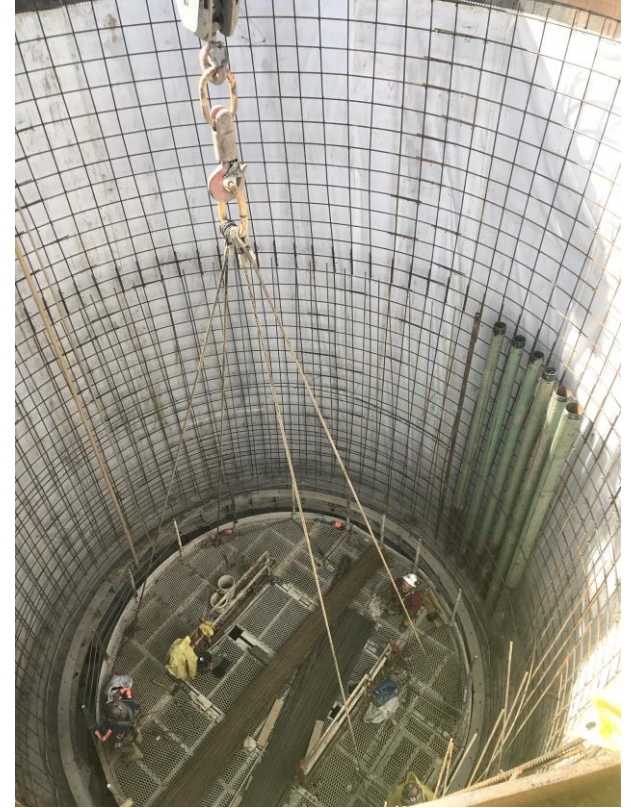
Shaft wall concrete preparations
