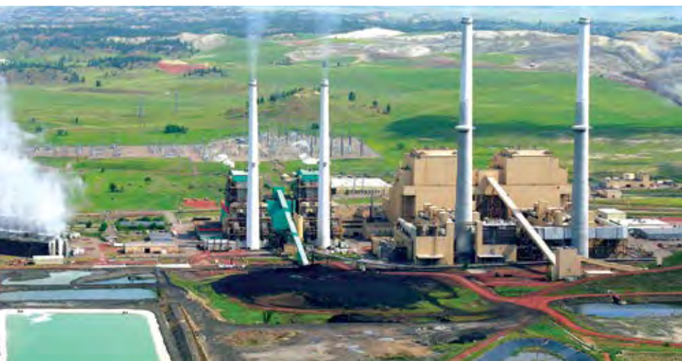
The Colstrip Generating Station will burn Rosebud's coal until at least 2025. (Photo: Puget Sound Energy)
