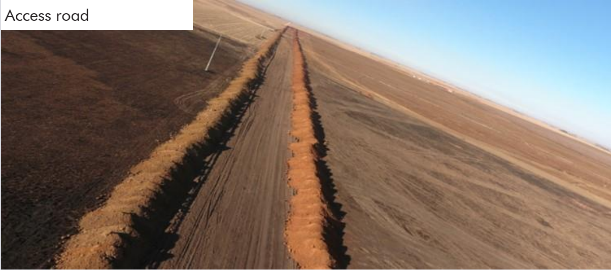
Box cut topsoil removal
