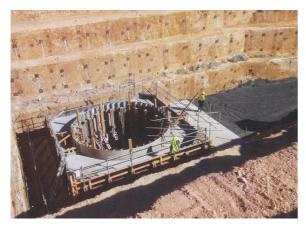
Shaft sub-brace concrete structure complete
