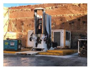
Raisebore on the fresh air intake/hoisting shaft collar
