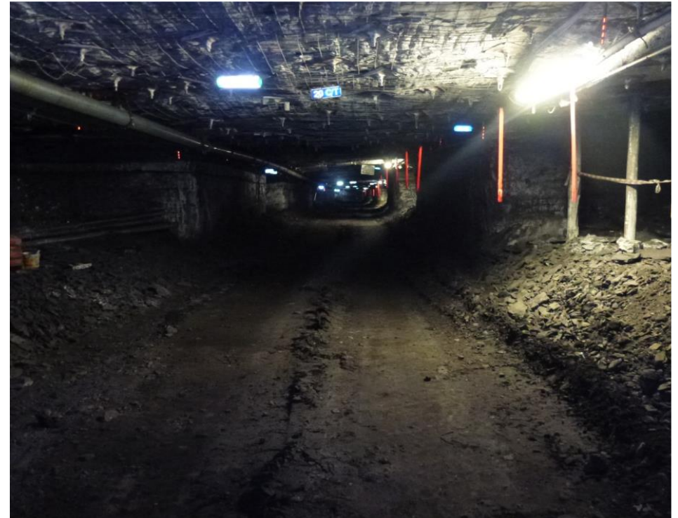
First development unit in place (above), with first coal cut late September 2019
