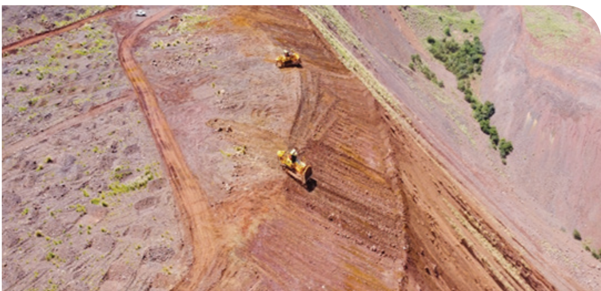
To improve safety, bulldozers undertaking potentially hazardous reshaping work at Thabazimbi iron ore mine are operated remotely.
