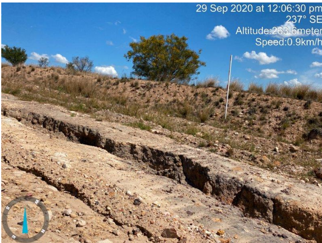
Photo 2: Erosion and sediment was generally very good. Area of erosion identified on the edge of an older haul road.
