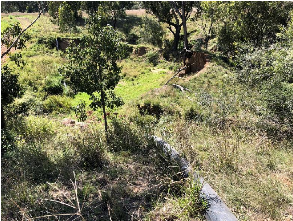
Photo 5: Saddlers Creek Offset - Monitor active gully erosion.
