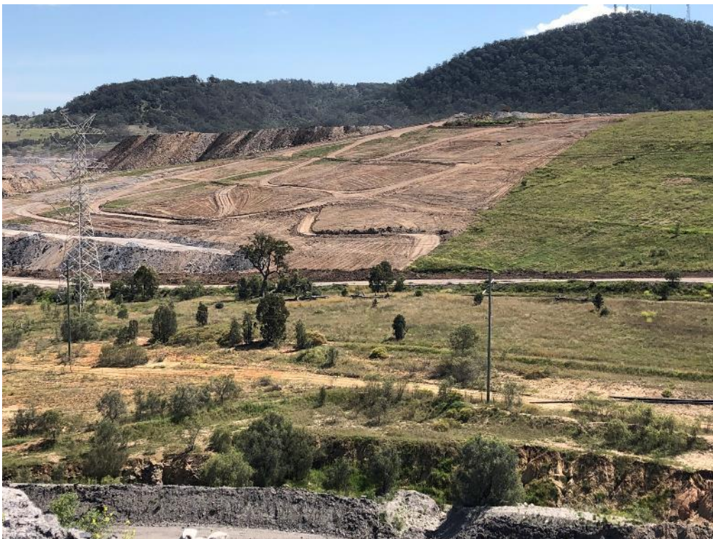
Photo 12: Saddlers North - Removal of existing rehabilitation for future dump space
