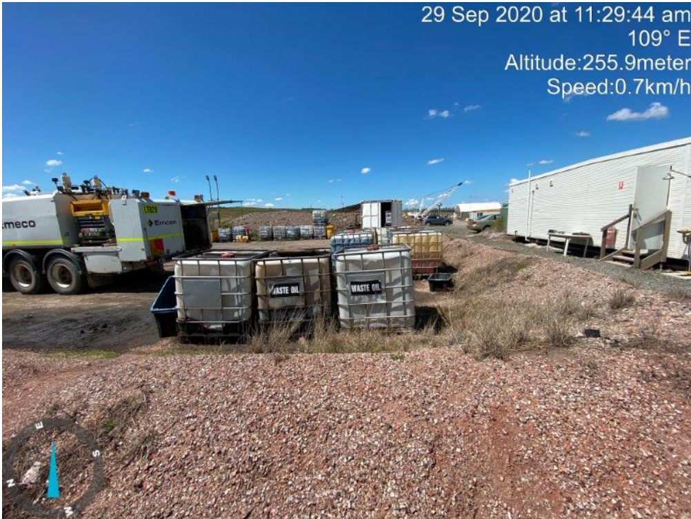
Photo 8: Waste oil not being stored within bunds in the contractor area.
