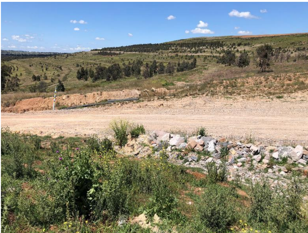
Photo 18: VD1 stabilising landform, good ground cover with contour banks stable with minimal sediment build up or failures. Continue to monitor and repair as required.
