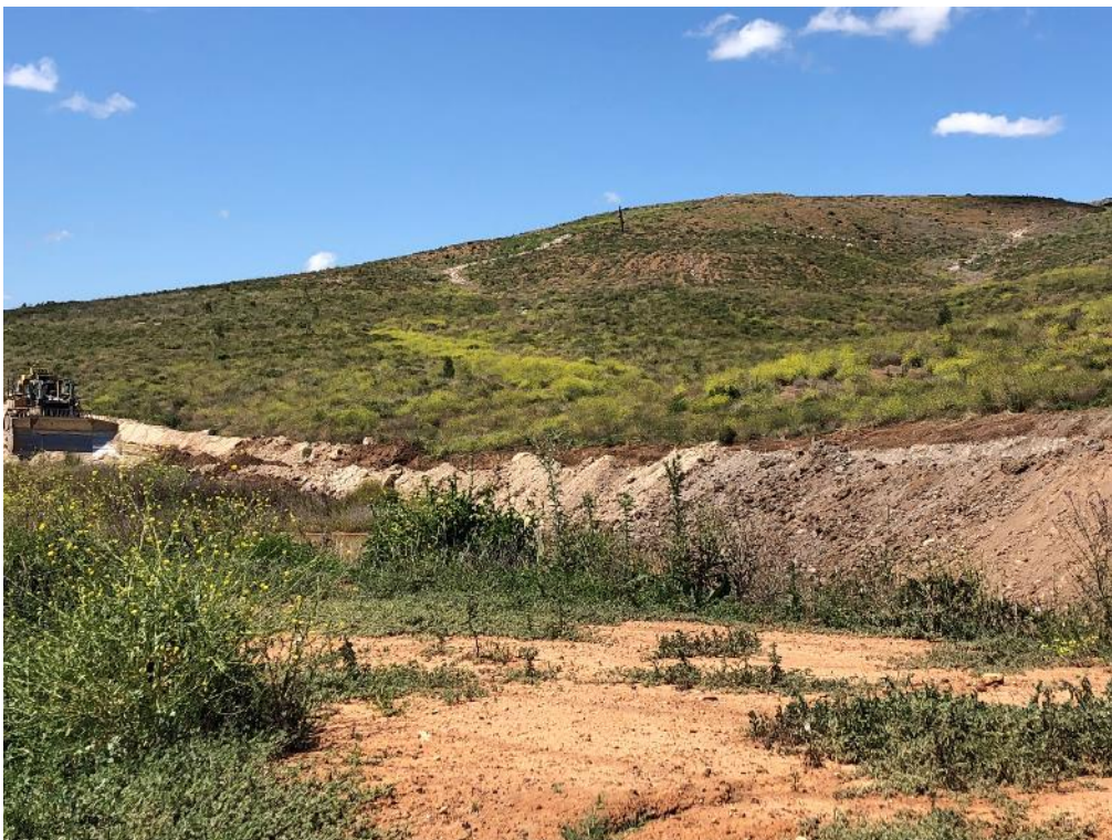
Photo 14: VD5 Soil surface and rehabilitation failure – implement planned re-rip and sow.
