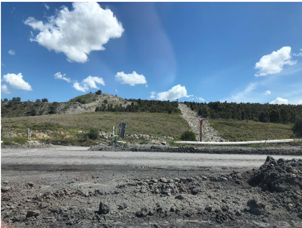
Photo 24: CD1 Drop structure appears stable.
