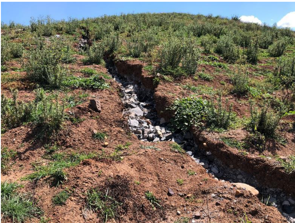
Photo 16: VD5 Gully erosion from dump crest bund failure – repair, contour rip and re-sow.
