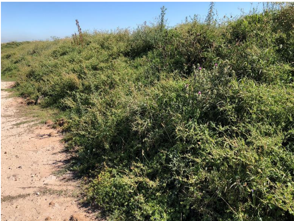
Photo 2: Drayton (CL229) Topsoil stockpile with evidence of weeds – requires treatment.
