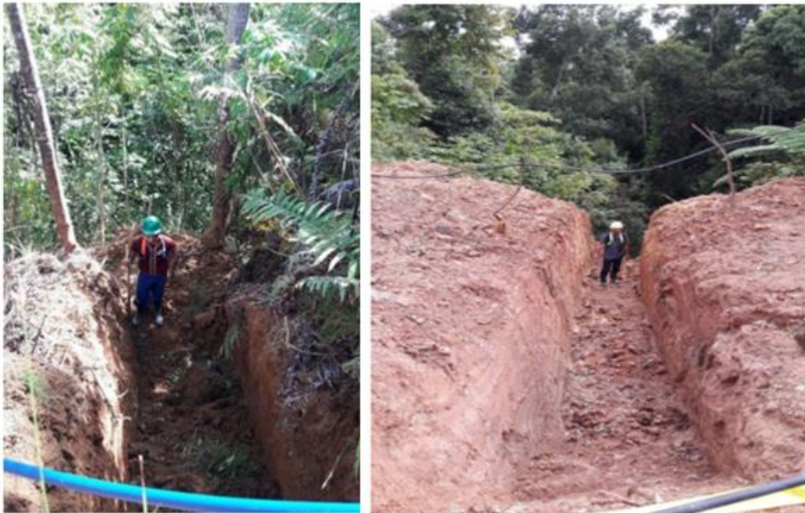
Figure 9-10: Trenches in South Miswi Area.
