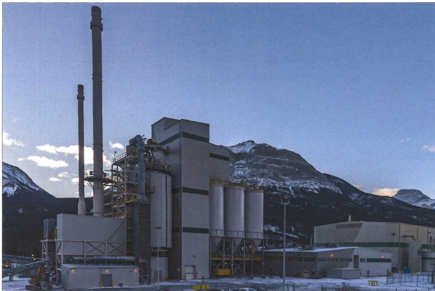
View of Plant: Preconstruction
