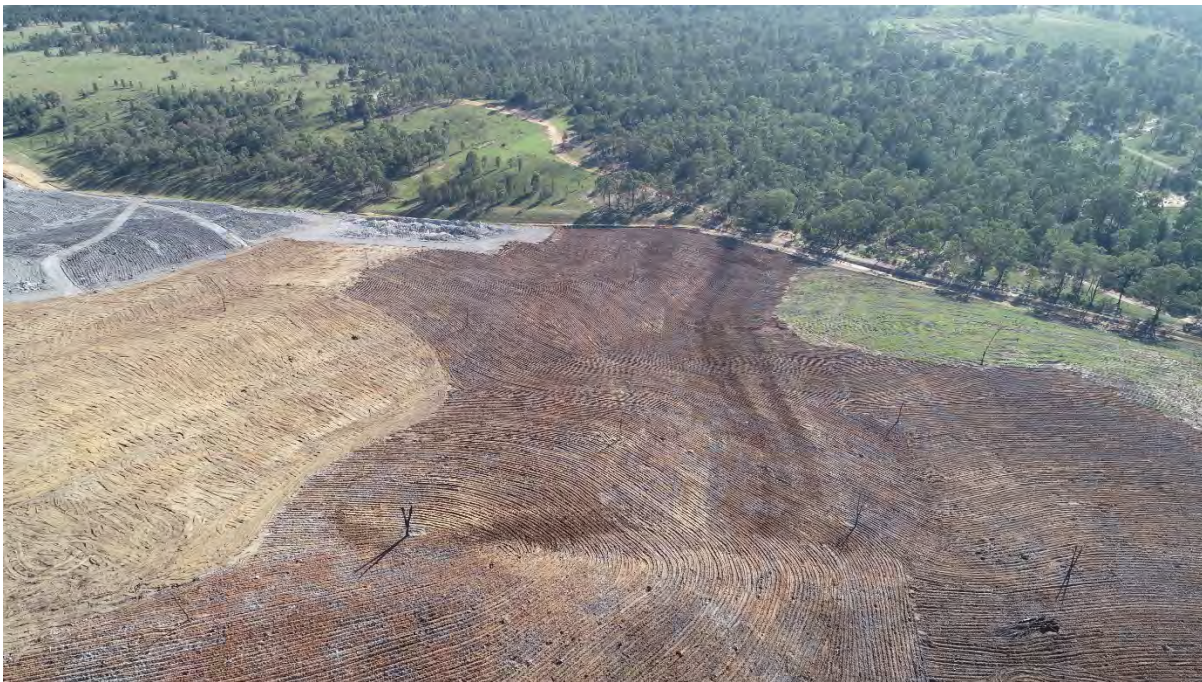
Photo 6 Built natural landform design surface, Eastern Placement Area Southern Dump
