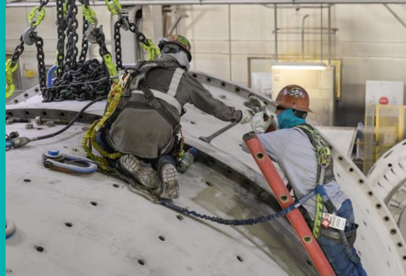
Ball mill shell #3 replaced. Increased reliability and throughput.
