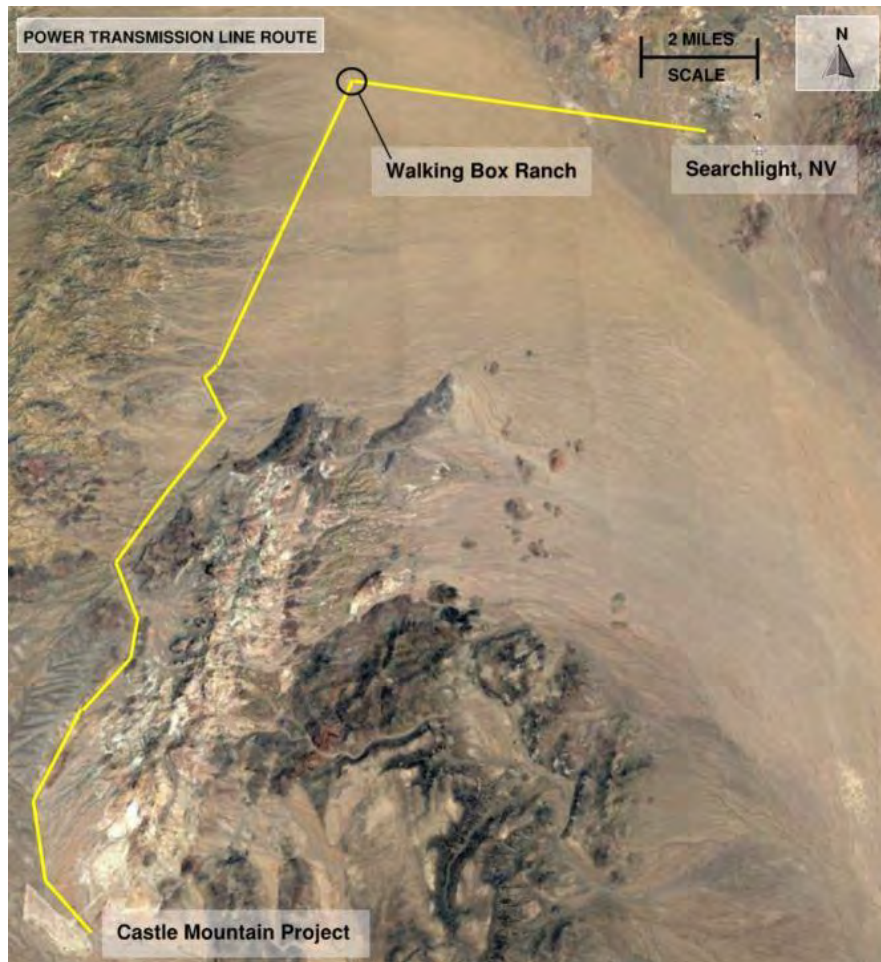
Figure 18-14: Power Transmission Line Route
