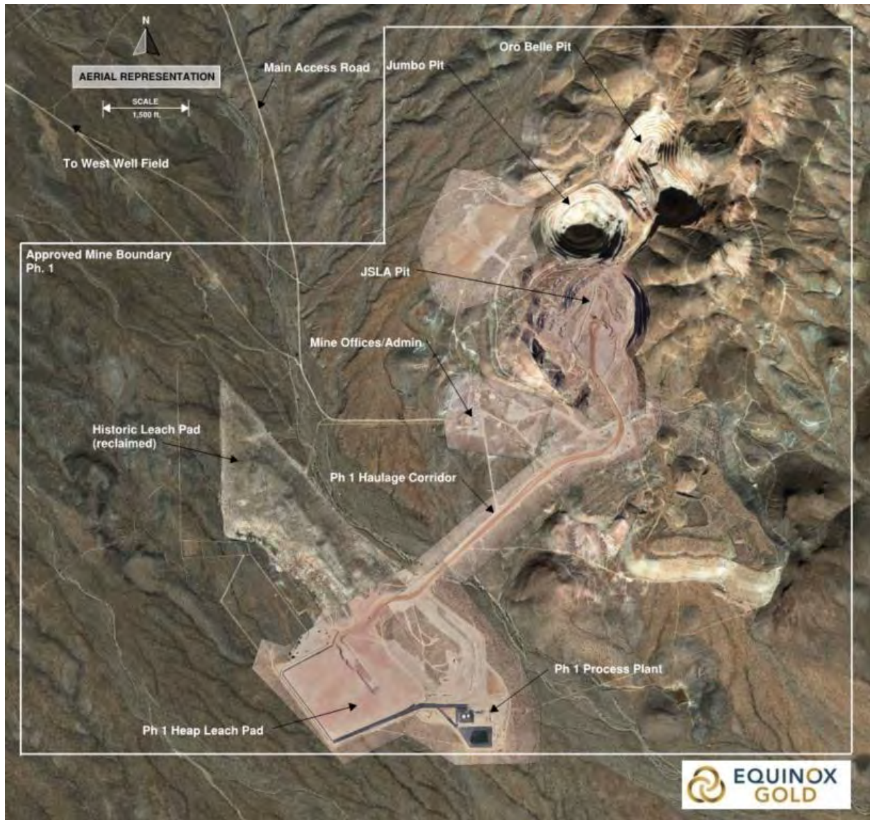
Figure 5-2: Site Infrastructure Map, Castle Mountain Mine (July 1 st , 2020 Representation)
