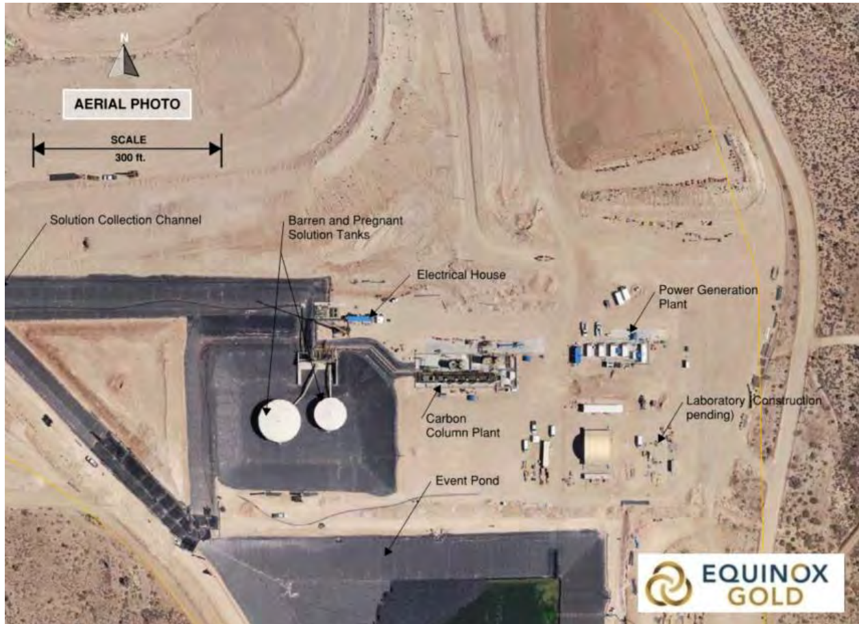
Figure 5-3: Castle Mountain Phase 1 Process Plant Aerial View
