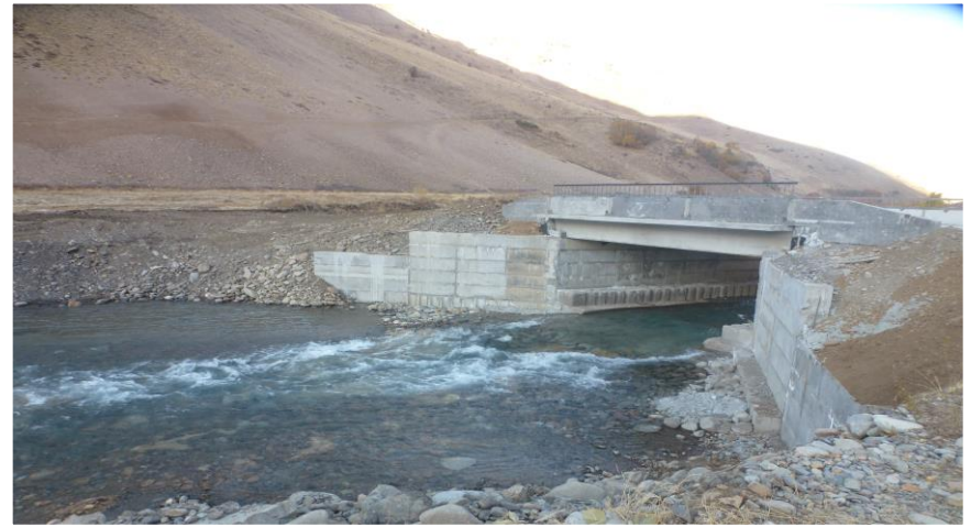
Lower Slipway Bridge
