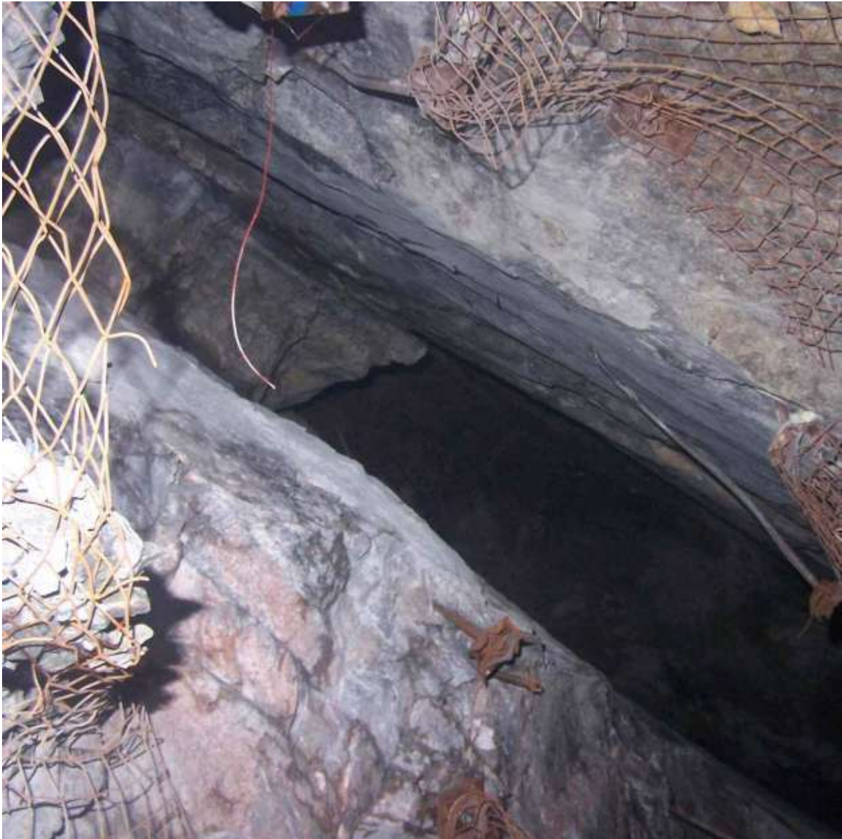
Figure 77. Stope (void) left after the ore has been extracted, showing the clean break along each side, and stable walls of the stope. Part of the remaining un-mined reef can be seen at the top left. Low-grade parts of the reef are left in place to act as pillars to support the surrounding ground (looking westerly).
