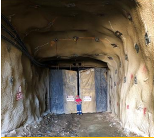
Entrance to underground
