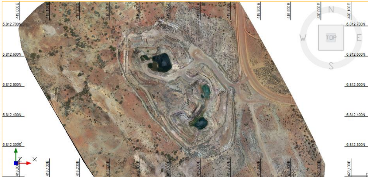
Figure 14: Aerial imagery of the historical Mt Marven open pit
