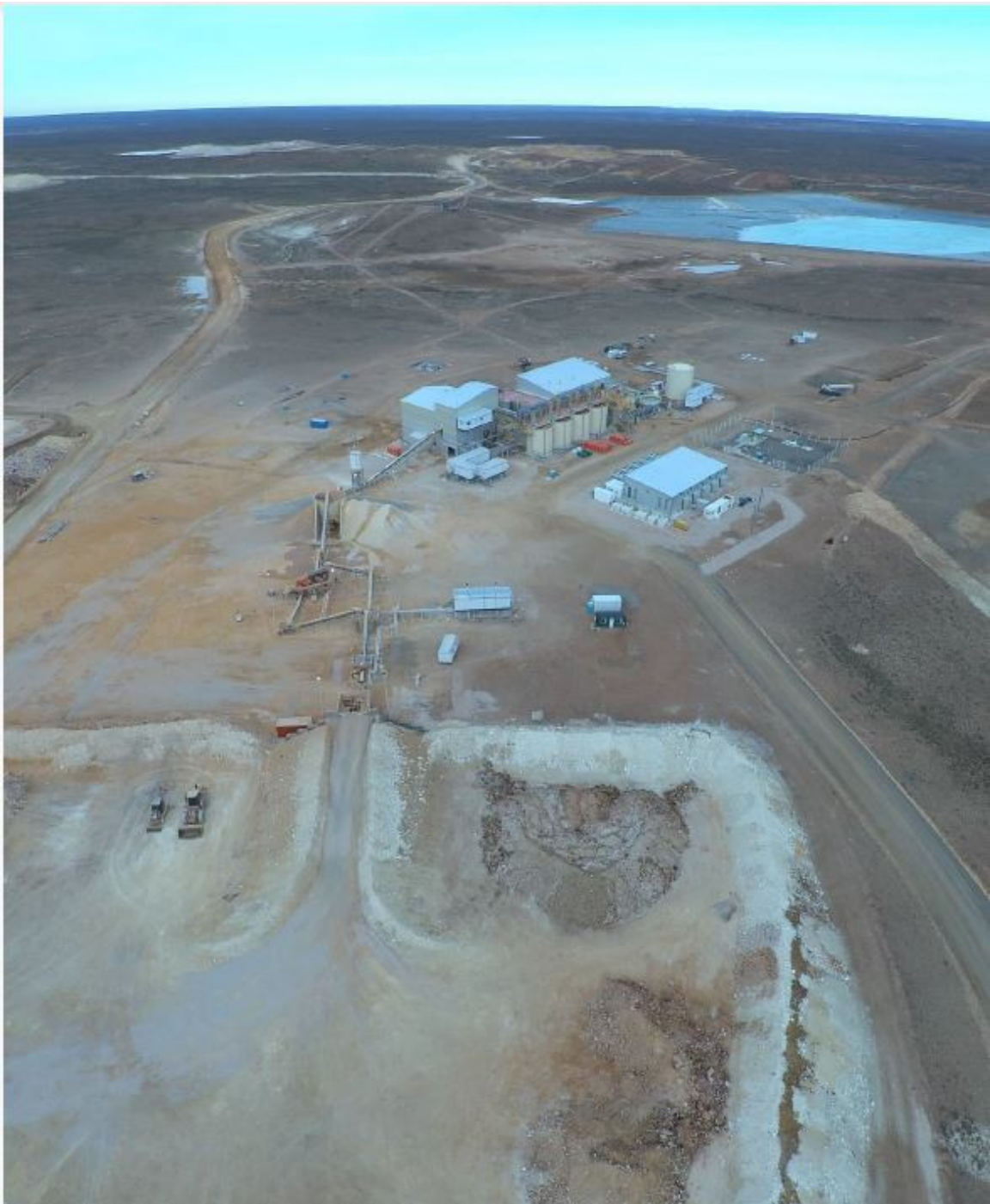
Figure 17.1: Aerial View of MDN Plant and Tailings Area at Martinetas
