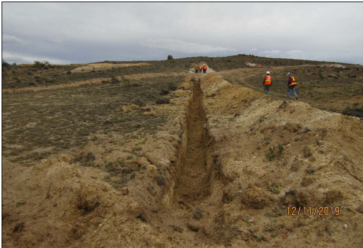
Figure 7.4: Trench Exposing Bedrock in the La Paloma Area
