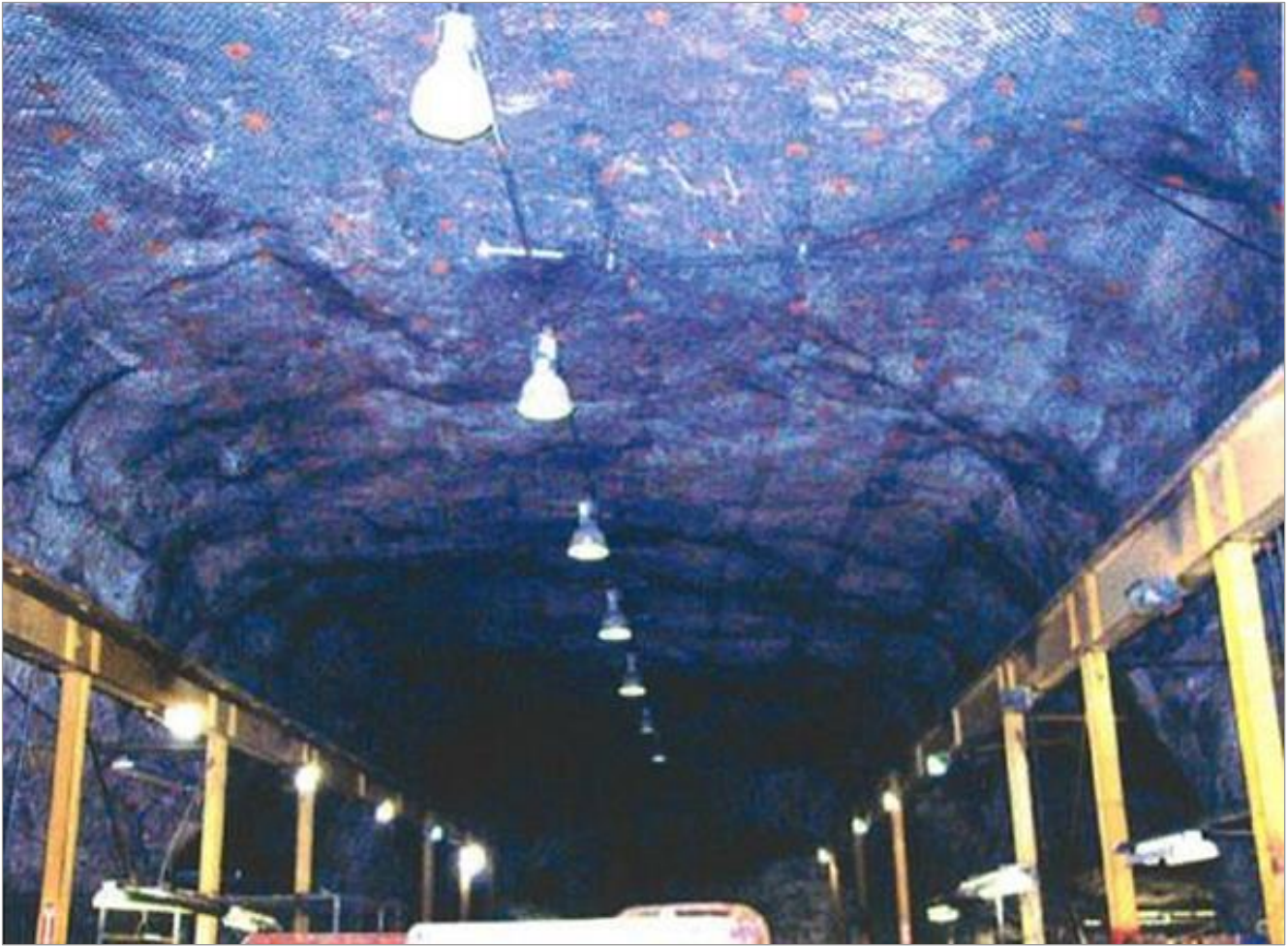
Figure 16.7 2,500 Level workshop ground conditions
