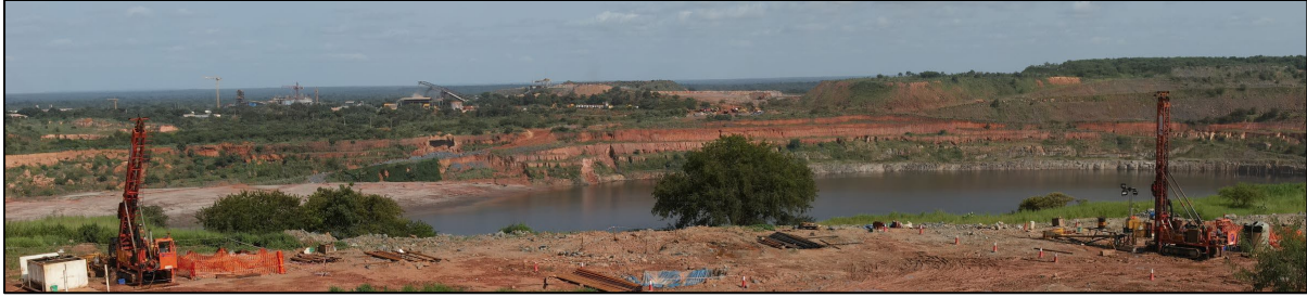
Drilling in progress at Morila NW
