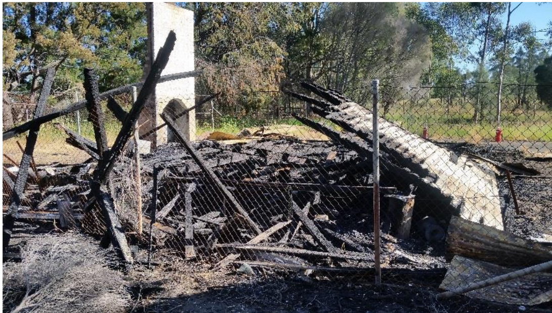
Figure 23: Demolition of Hebden PS - before
