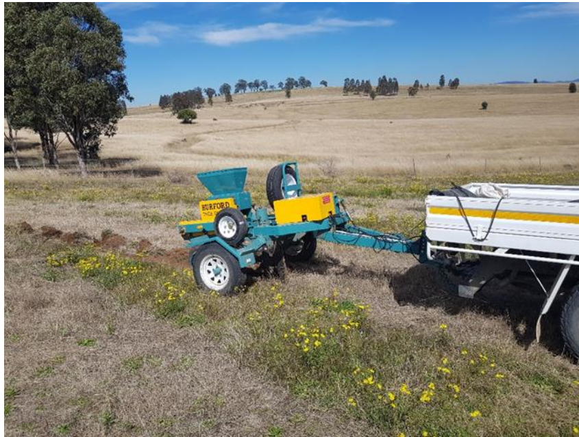
Figure 13: Example of direct seeding works completed at Stringybark Offset Area
