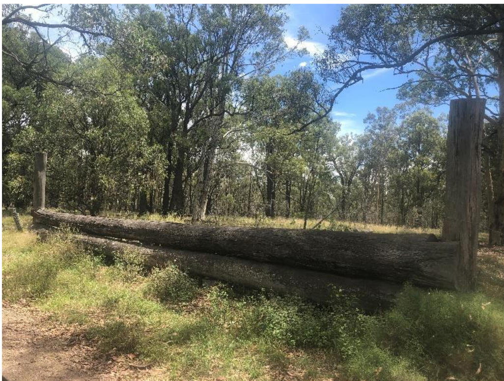
Figure 22: Timber loading ramp to be managed in-situ
