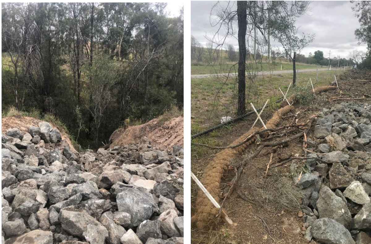
Figure 29: Yorks Creek Diversion (Hebden Rd) remediation works completed in 2020
