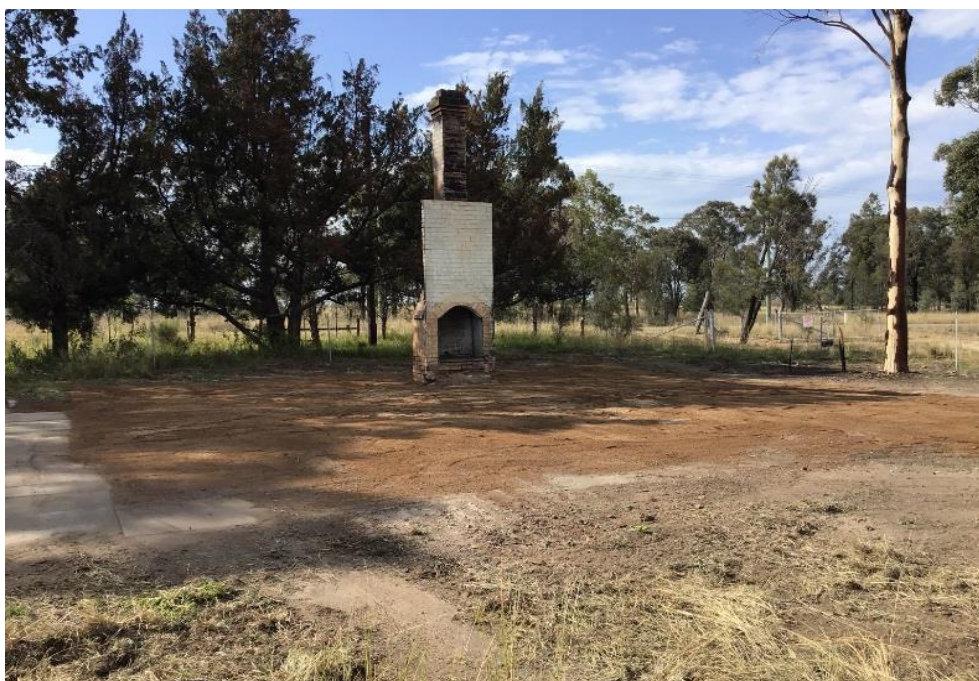
Figure 24: Demolition of Hebden PS - after
