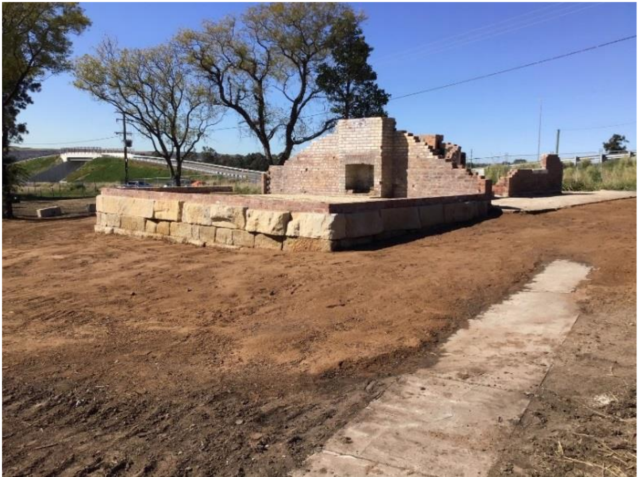
Figure 26: Demolition of Ravensworth Public School - After
