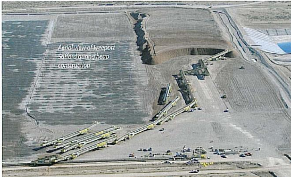
Figure 14-9: Grasshopper conveyors and stacker
