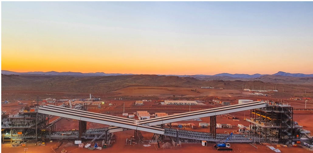
Ore processing facility
