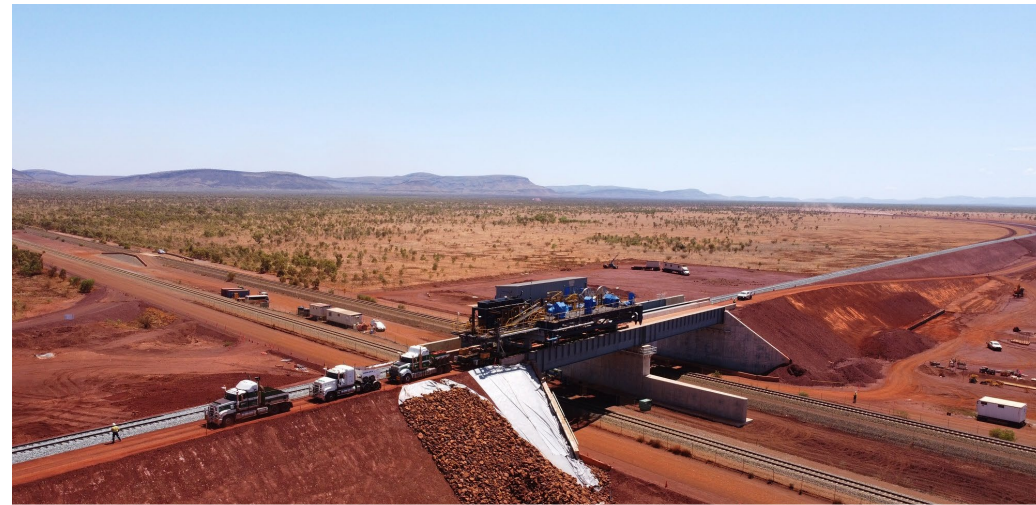
Eliwana rail bridge
