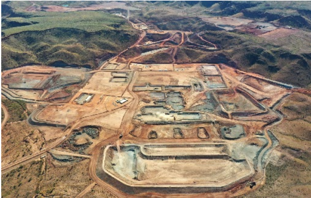
Ore processing facility site
