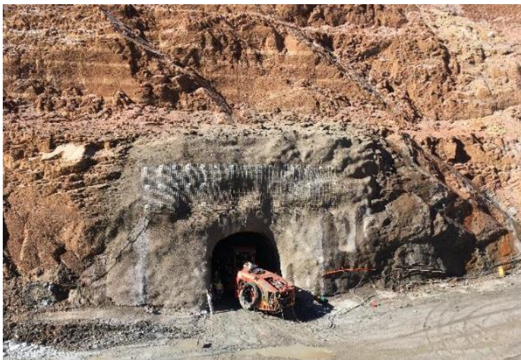
Jumbo working in Moonbeam portal Friday 6 th September
