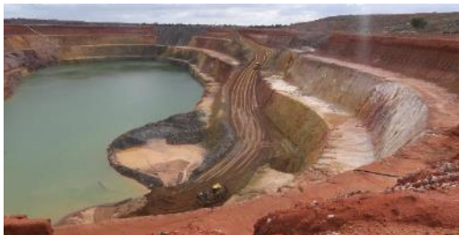
Building the ramp to start dewatering 16 th June
