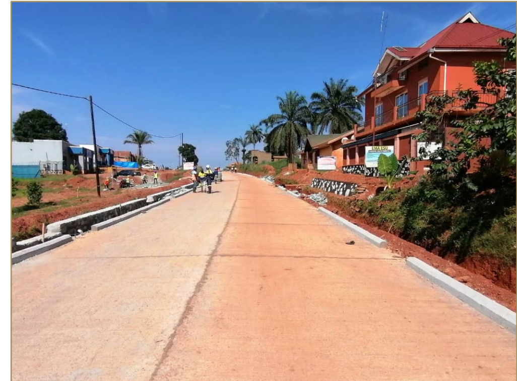
Construction of the concrete road in Durba
