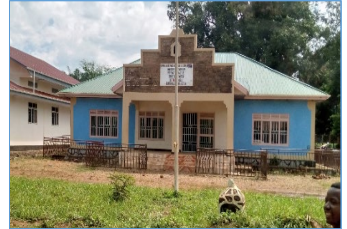
Renovation of Surur Admin Office
