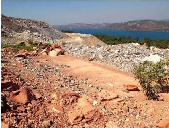
Plate 7-2: Accumulation of sediment in catchment berm (2015)
