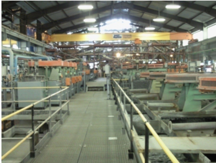
Figure 16.7: General view of flotation cells in Merensky plant.
