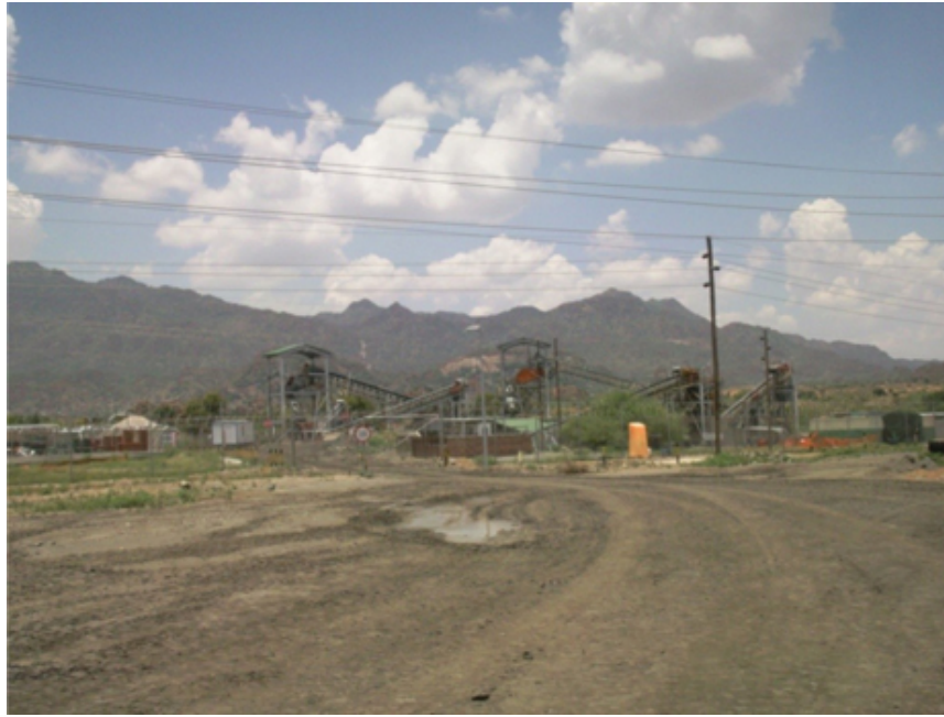
Figure 16.12: General view of the UG2 crushing facility.
