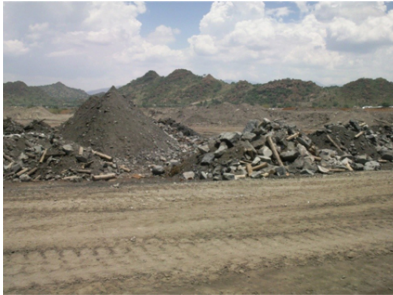
Figure 16.9: Removed oversize rock and support timber.
