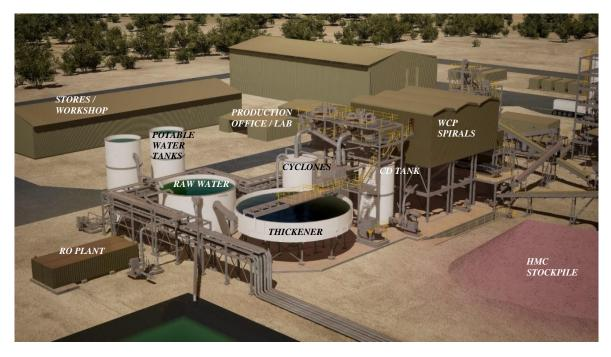
Figure 5 Lucky Bay Garnet Mine Wet Concentrator Plant
