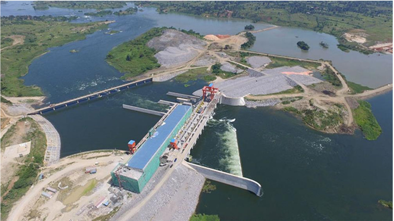
Figure 24: Isimba hydroelectric dam with 183 MW installed capacity.
