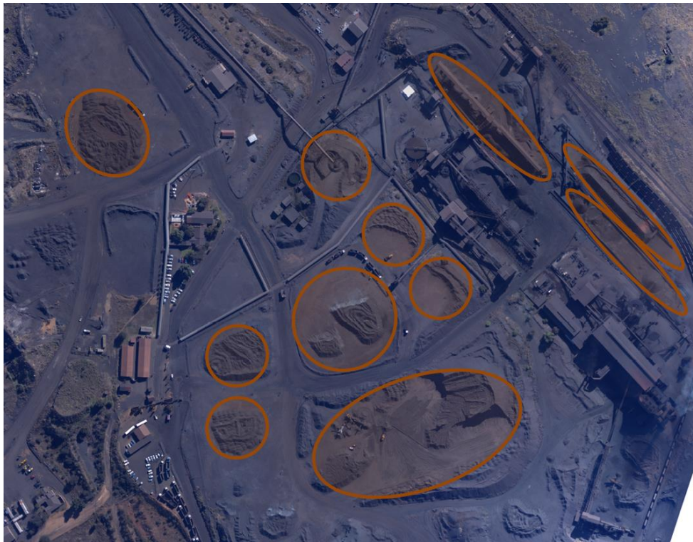
Figure 3.4-2 Aerial photograph indicating gantry and dumping type stockpiles.
