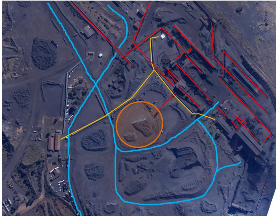
Figure 3.4-1 Aerial photograph indicating personnel access, hauler routes and conveyors at Mamatwan Plant. The blue lines are indicative of hauler routes, while personnel access the plants via walkways indicated in yellow. Stationary conveyor systems indicated are indicated with red. Road-transport load-out area with its road-hauler-weigh-bridge is indicated with.
