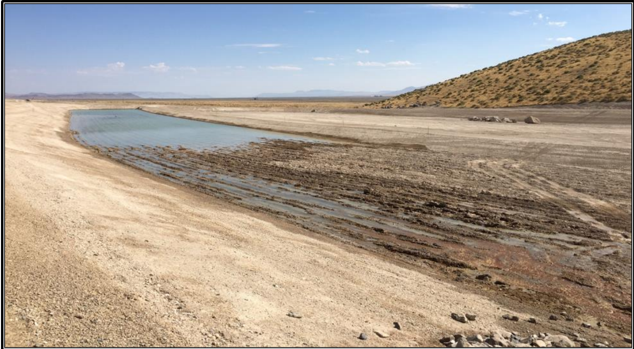
Figure 18-4 Rapid Infiltration Basin During 2017 Pump Test
