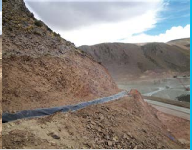
Waterproof canal at the mine
