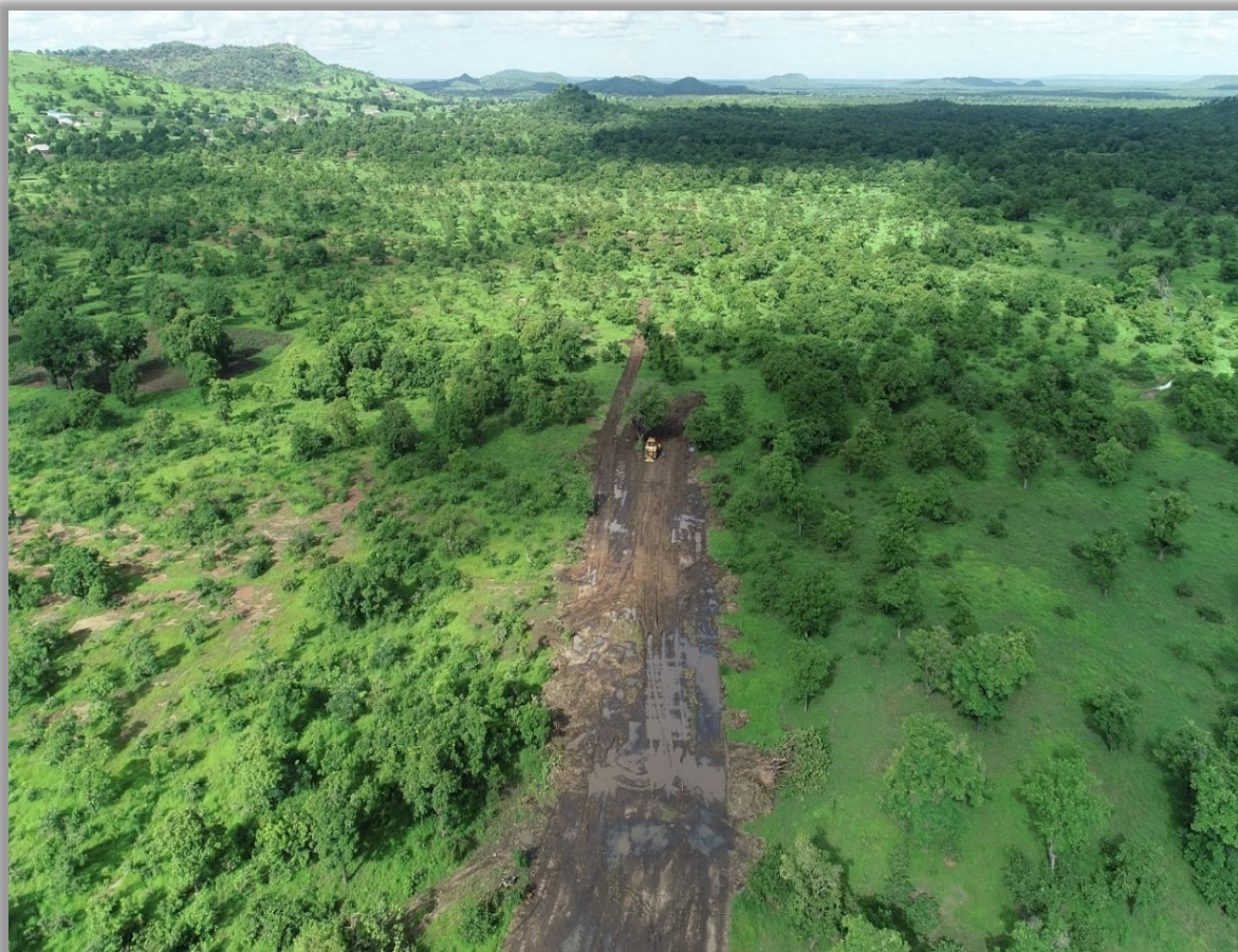
Figure 3 – Progress of Namdini Clearing for the Pioneer Access Road
