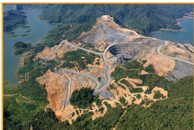
Above: An aerial view of the Ban Houayxai Gold-Silver Operation showing the Colluvium North, Colluvium South and open-pits
