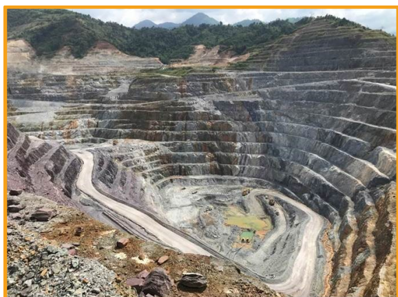
Above: Mining of high grade ores in the Phu Kham Copper-Gold Operation open-pit bottom stage 6
