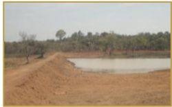
Tongon Low Capacity Dam
