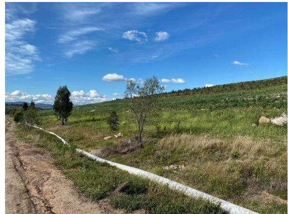
Photo 4 – Remediation works undertaken during 2020 across lower Western Emplacement Area slopes
