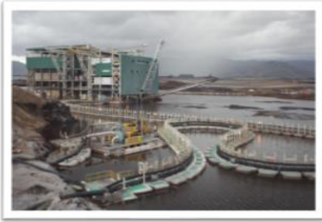
Dredging at front of the pond
