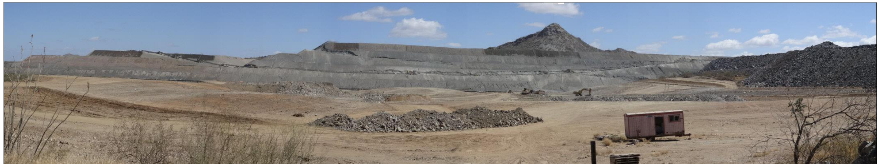
Figure 17.8 Heap Leach Pads as Viewed from the Road to the La Chicharra Pit with Phase 6 Under Construction in the Foreground (May, 2017)
