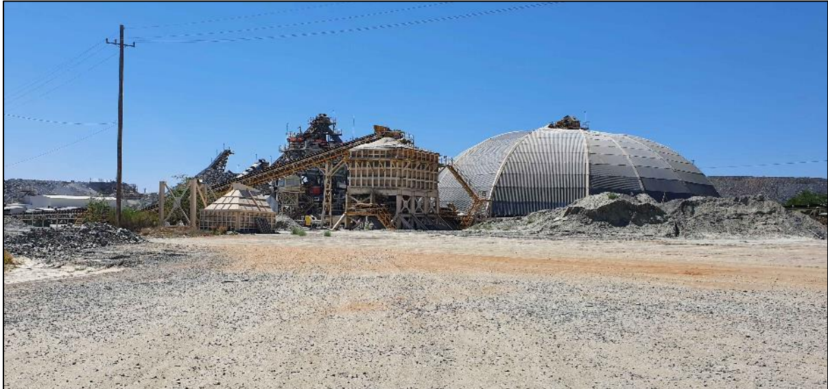
Figure 12.6 Partial View of the Crushing Facility
