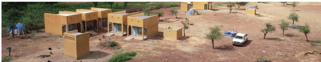
New homes under construction for affected people
