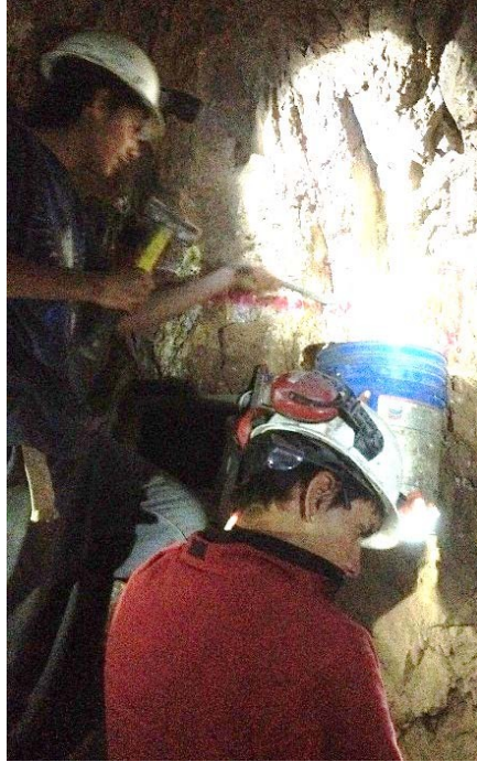
Figure 11-2: Channel Sample Collection
