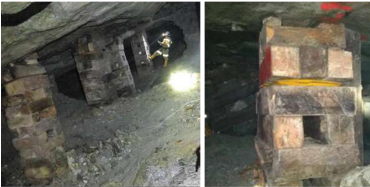
Figure 16-7: Timber Packs Example Used by Segovia
