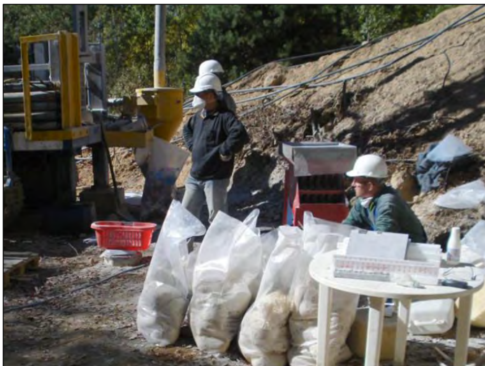
Figure 27. RC Samples lined up at the rig with riffle splitter and cyclone located in the background
