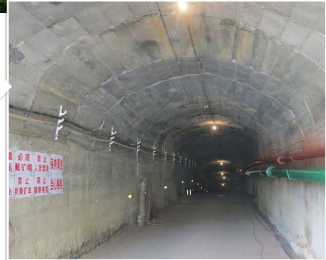
Main Access Ramp
