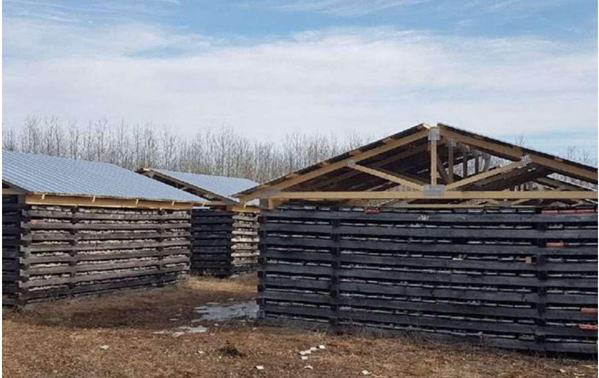
Figure 11-64: Secure core yard storage
