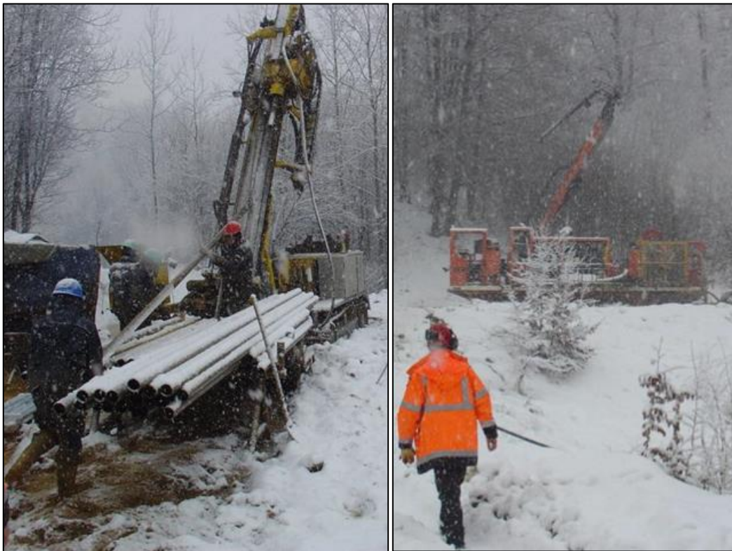
Figure 10.1 – Diamond (left) and RC Drilling (right) at Bigar Hill
