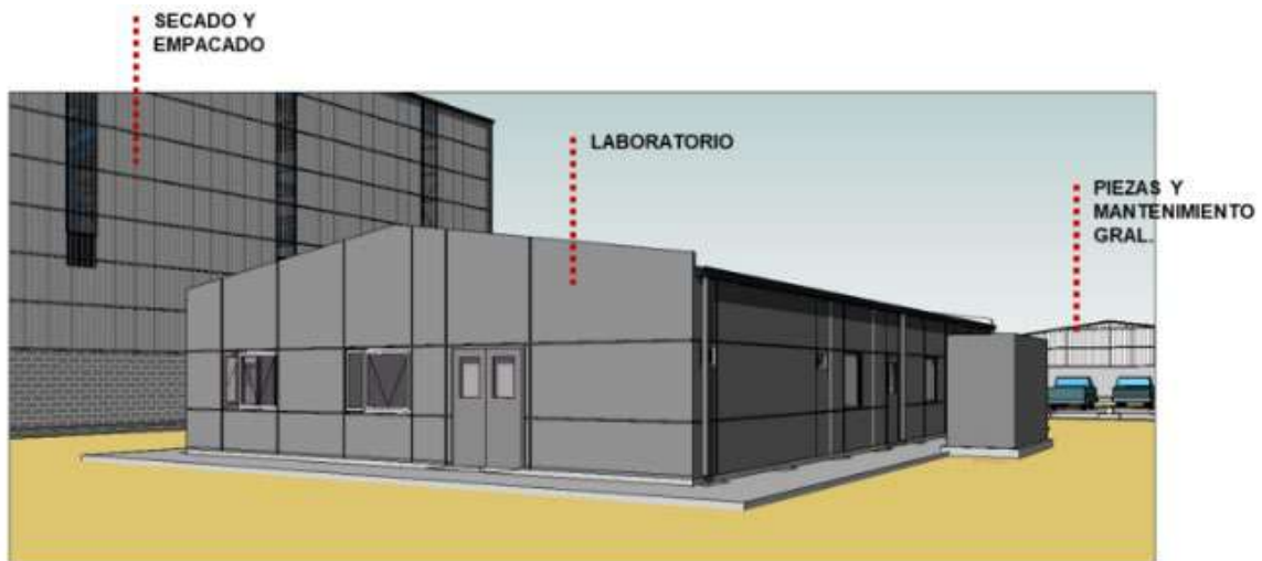
Figure 18-10: Fiambalá site – laboratory building.
