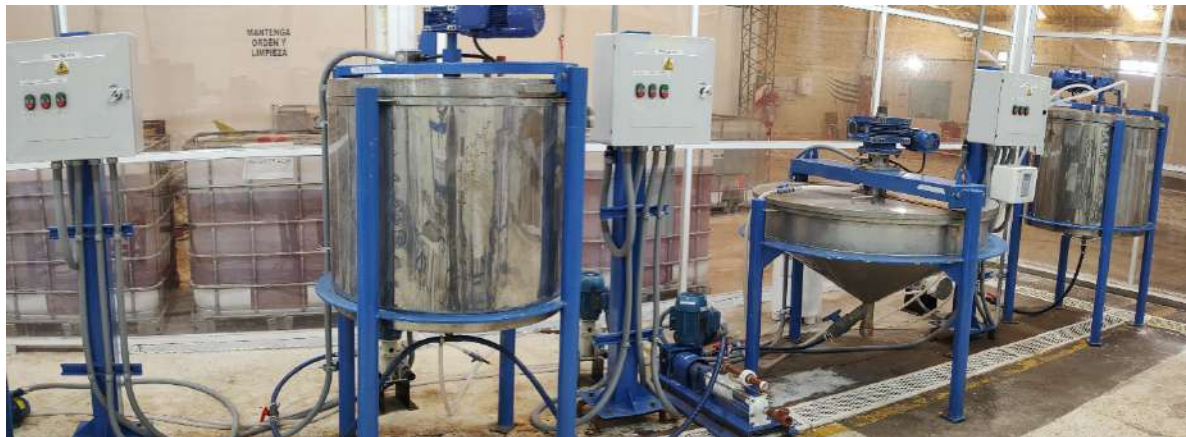
Photo 13-8: Equipment used in stage tests.
