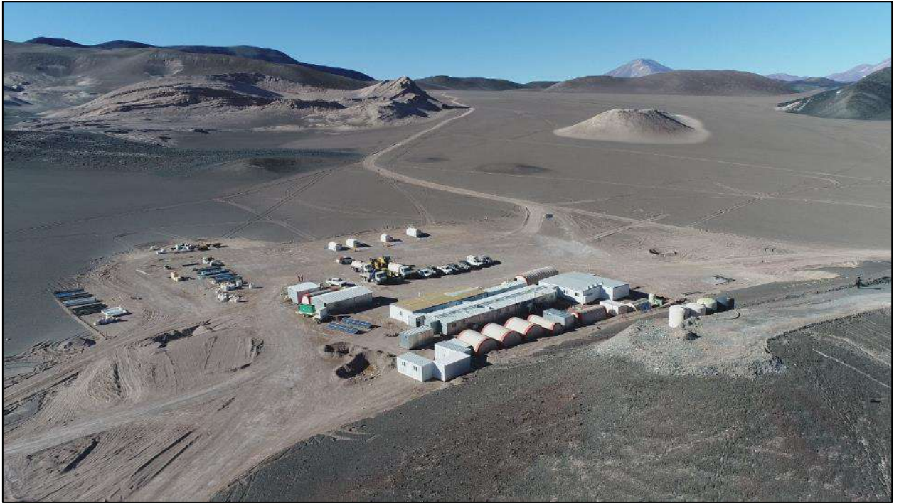
Photo 4-3: View of the 3Q Project Camp.
