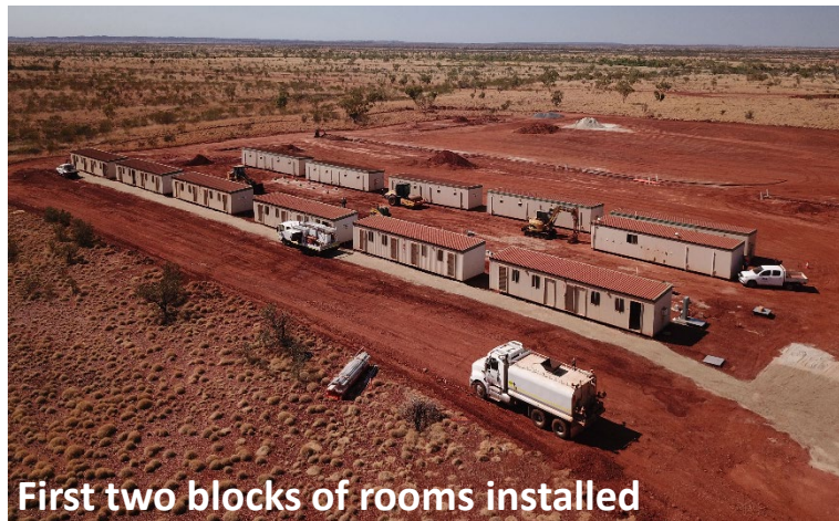
240 room village starts installation
