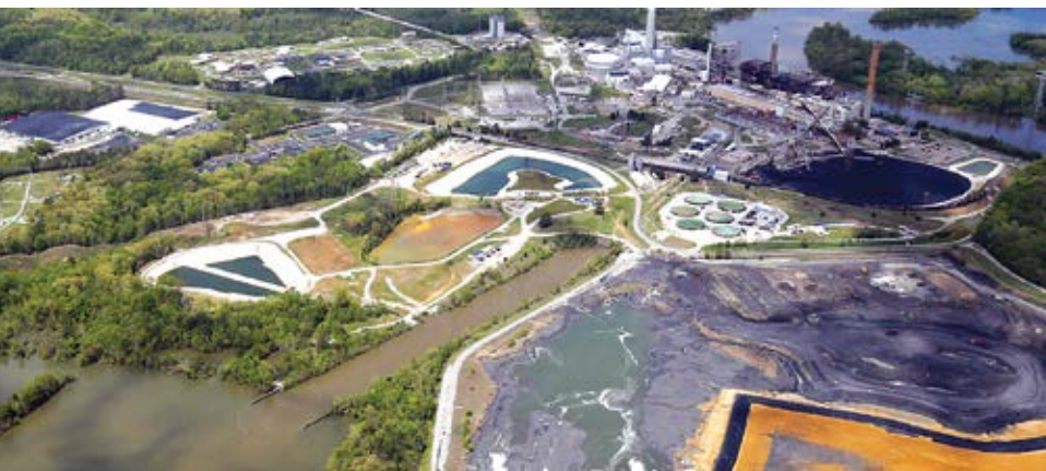
The Chesterfield power station (above) has been ordered to remove 15 million yd 3 of coal ash.
