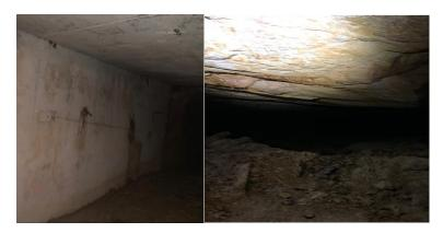
Image 5: Good conditions reported of the Qala Adit shaft infrastructure (left) and the K9A hanging wall (right)
