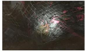
Hoisting shaft Leg 1, raise-bore pilot-hole break-through on target at the mid-shaft access
