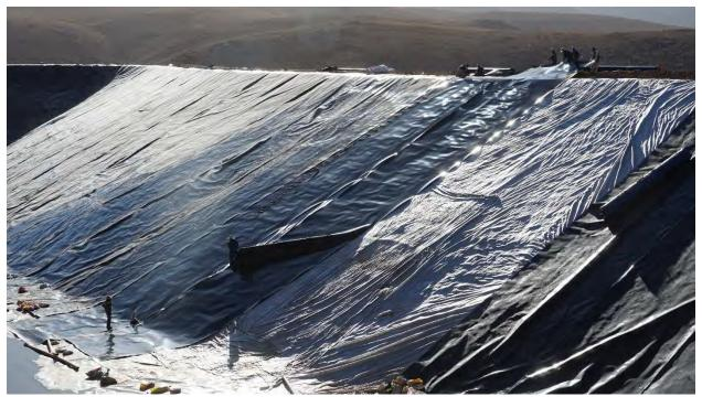
Figure 2: Installing the liner on the 60,000m<sup>3</sup> water retention basin
